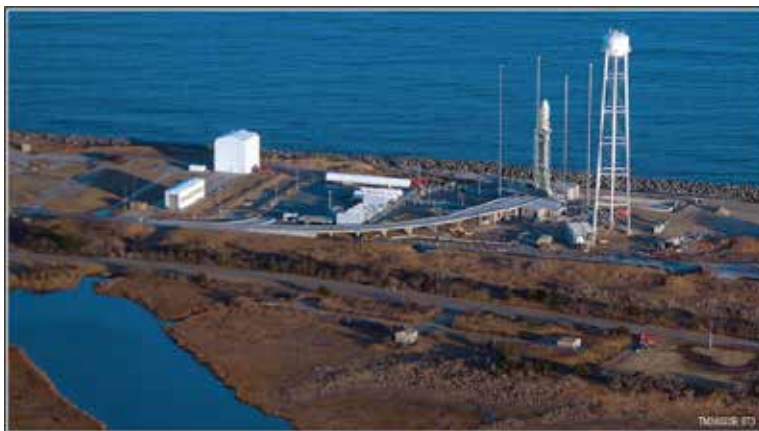
Figure 7.2.2.1-1. WFF Launch Pad 0A
