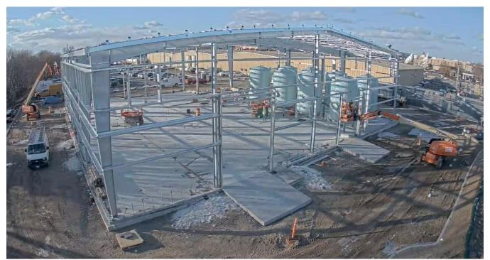
**Treatment System Construction Progress:** We are making very good progress on the construction of the RW-21 treatment system building. The exterior steel structure is nearly installed as are eight carbon filtration tanks. (Aerial image today).
