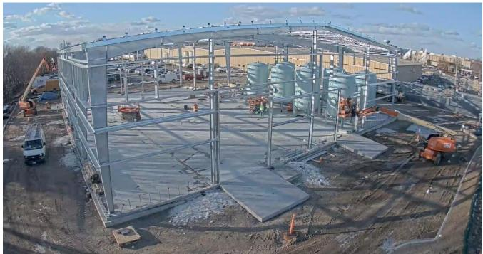
**Treatment System Construction Progress:** We are making very good progress on the construction of the RW-21 treatment system building. The exterior steel structure is nearly installed as are eight carbon filtration tanks. (Aerial image taken Jan 10).
